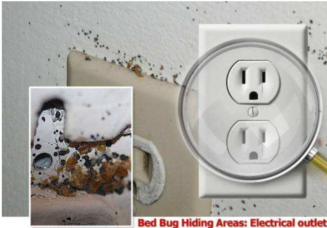
Bed bugs around electrical outlets Stop bedbugs.com
